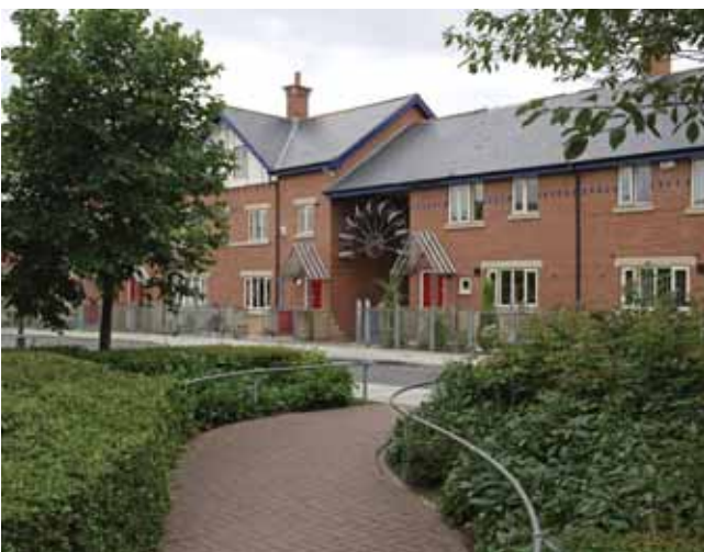
St John's housing development, off Marton Road
