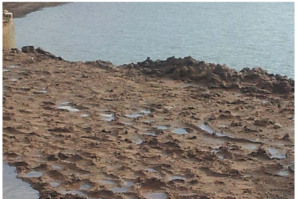
SuDs work takes place in Middlesbrough
