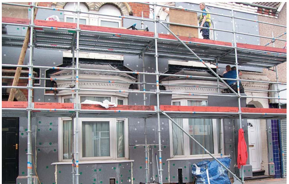
External cladding work takes place
